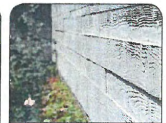
Fish Sorting Channel Board Form Concrete
